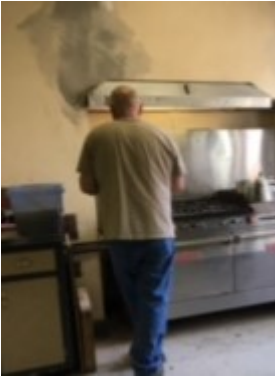
Jim Cherry getting the walls ready to paint. Lots of cracks to fill and smooth
