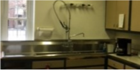
The new triple sink..... and primed walls!
